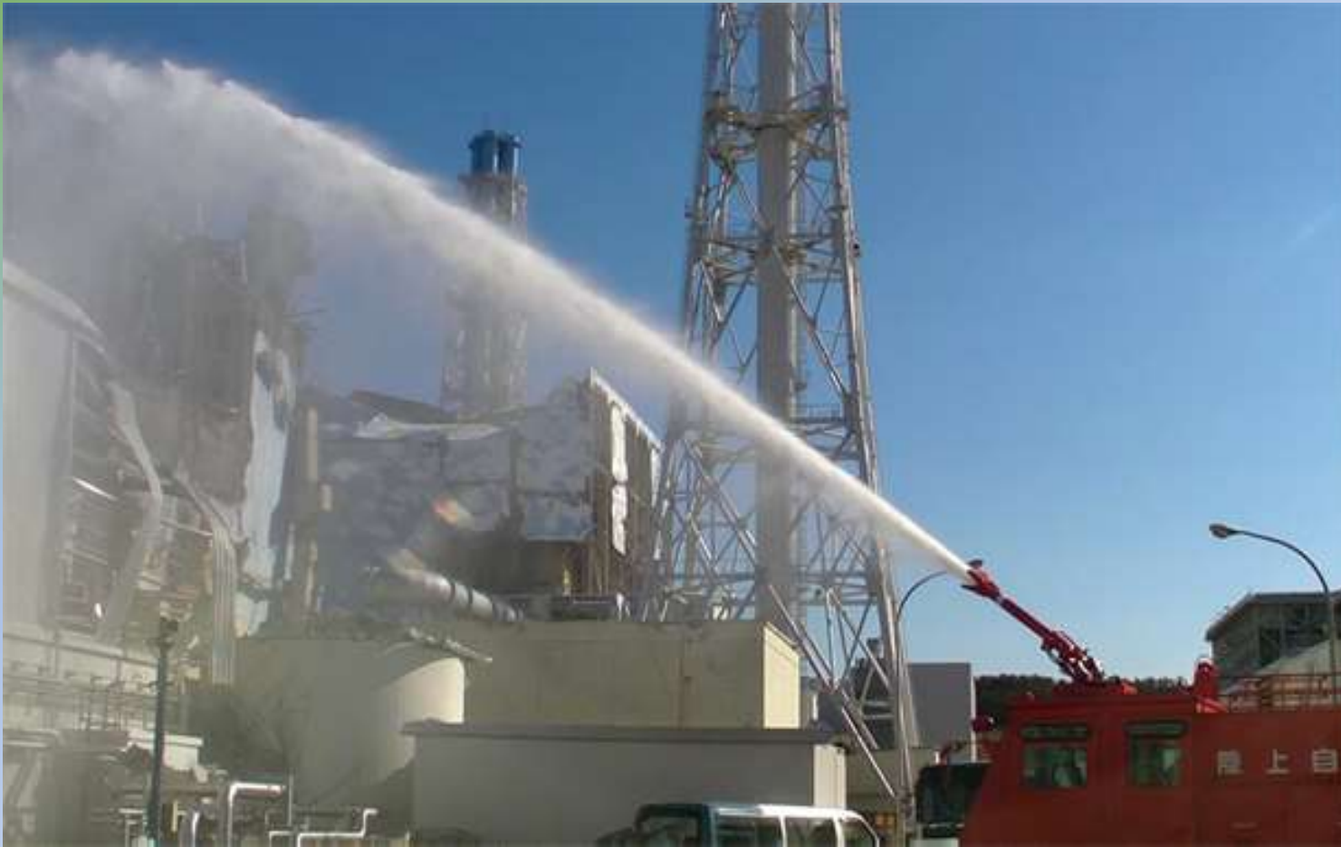
Injecting water into Unit 3 of Fukushima NPP.
